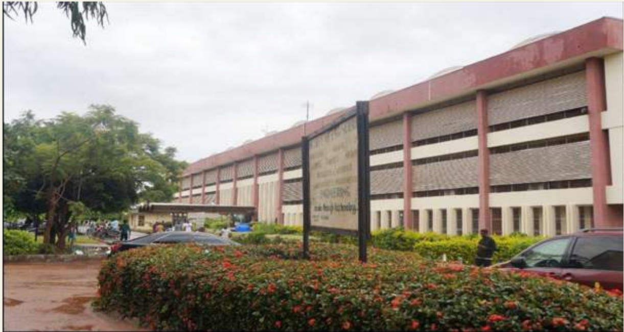
Consultancy for Rehabilitation of Ashim Ibrahim Library , Ahmadu Bello University, Zaria.
