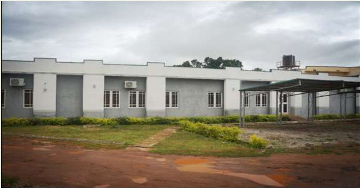
Construction of Radiology Unit Ahmadu Bello University Medical Centre, ABU Zaria.
