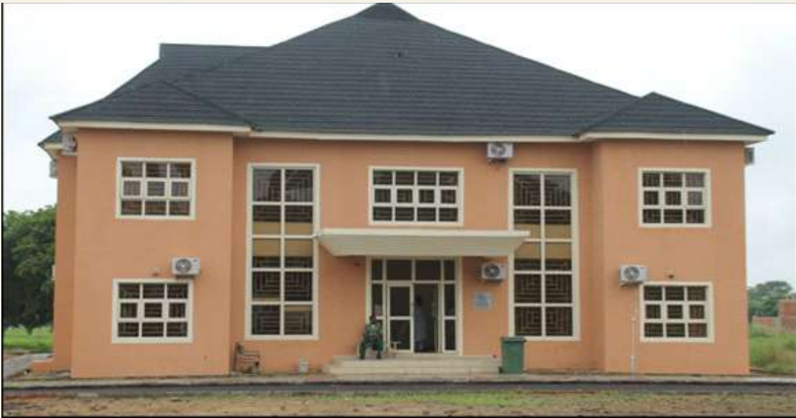
Design and Construction of National Farmers Helpline Centre (E-Extension Centre)
