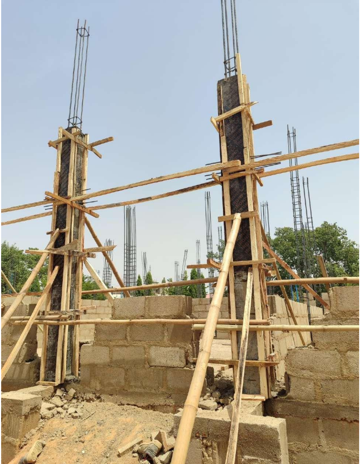
Form work for Column
