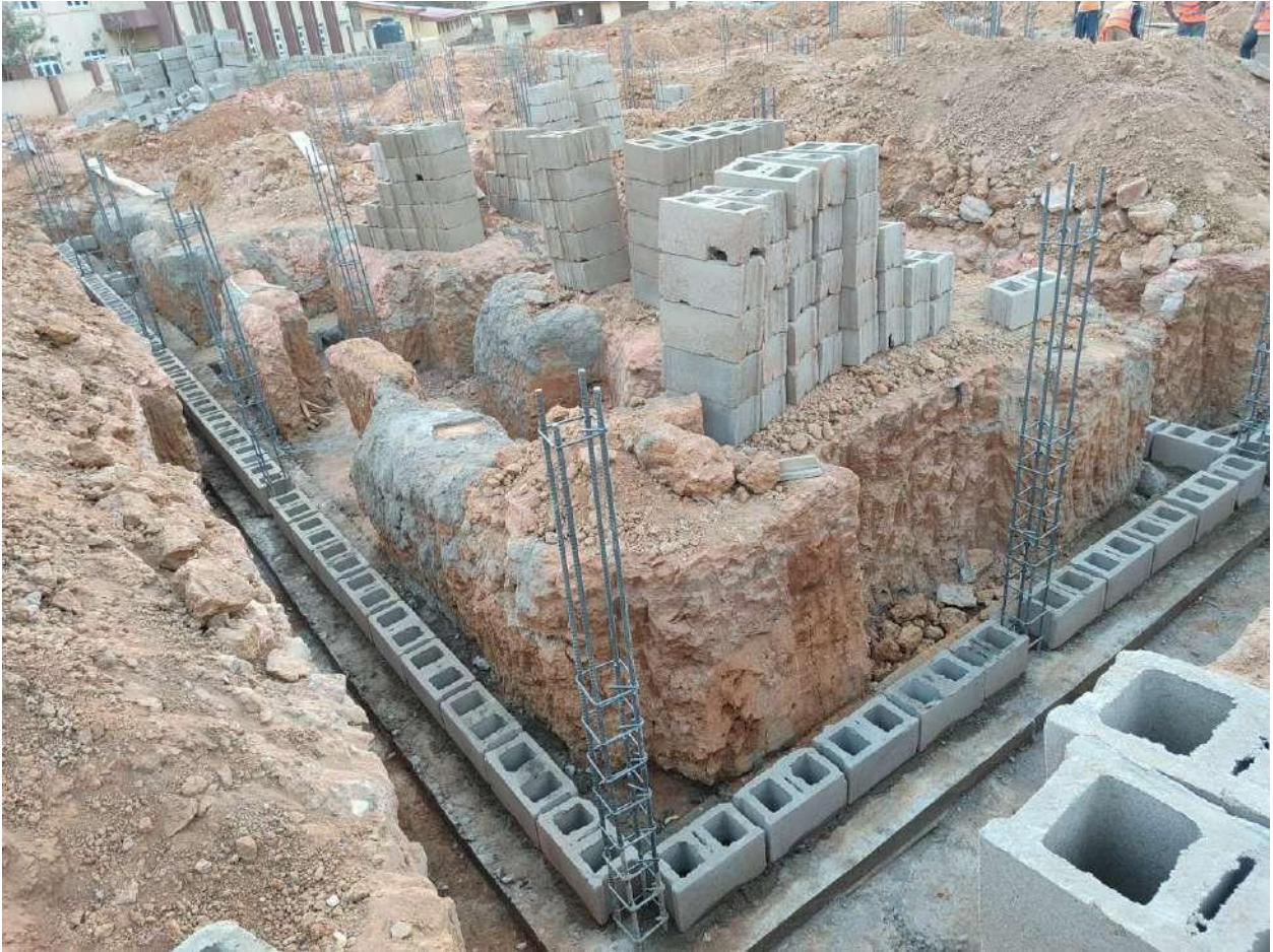
Block work in foundation
