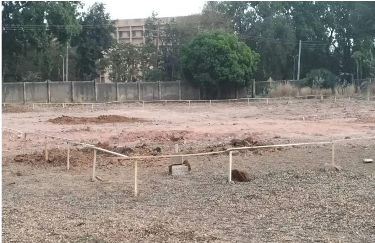
Building setting out
