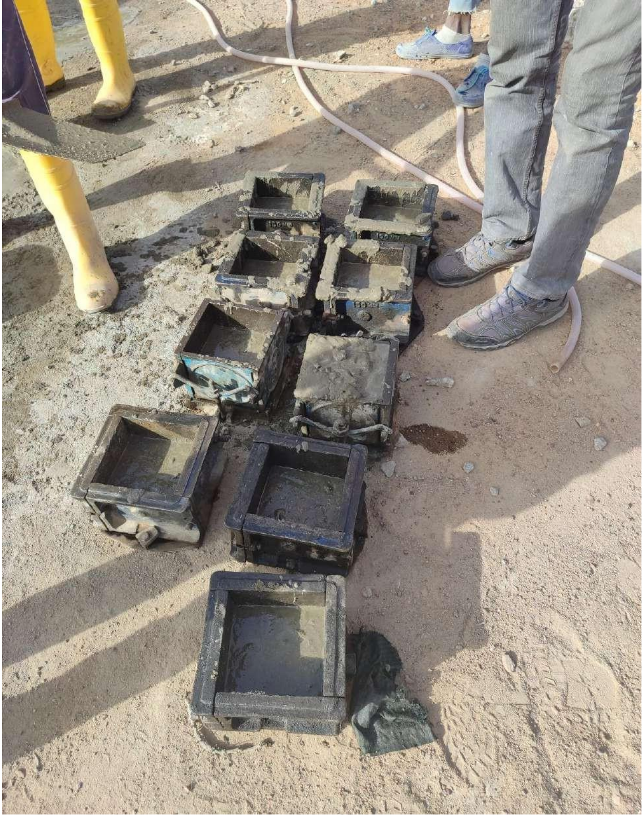
Casting of test cubes from Concrete for columns
