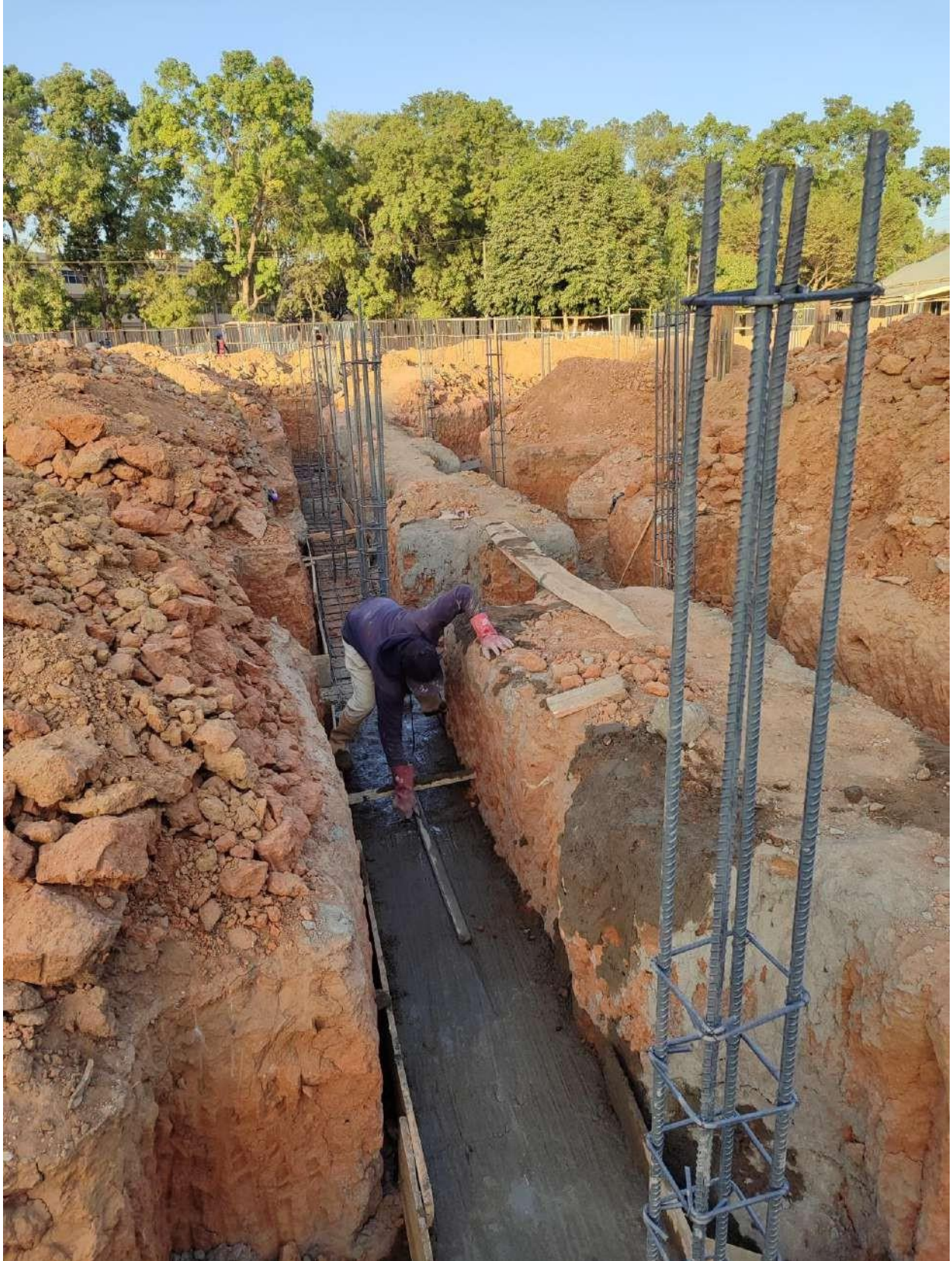
Formwork, reinforcement and concrete for Reinforced Strip foundation
