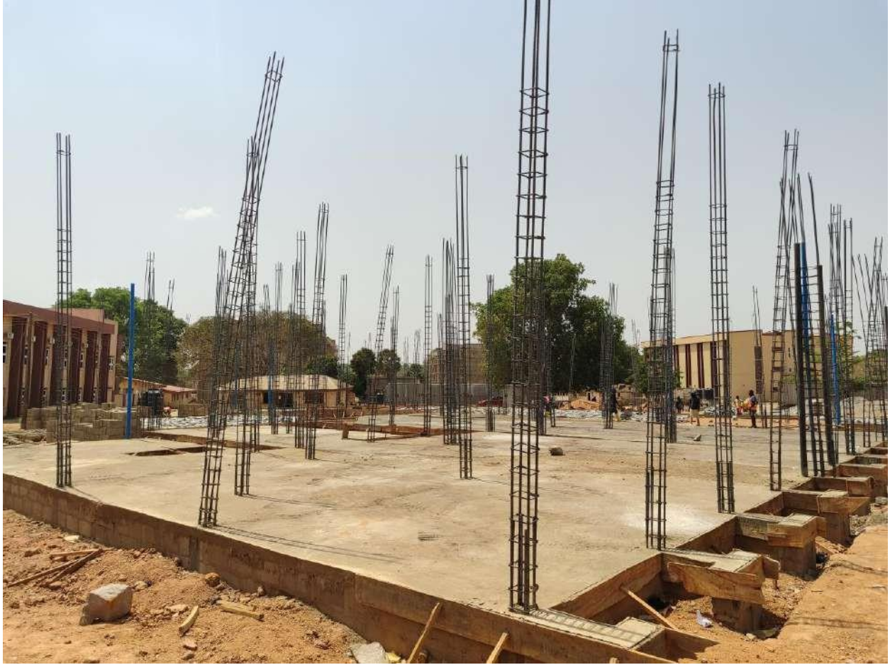
Completed section of Dam proof course
