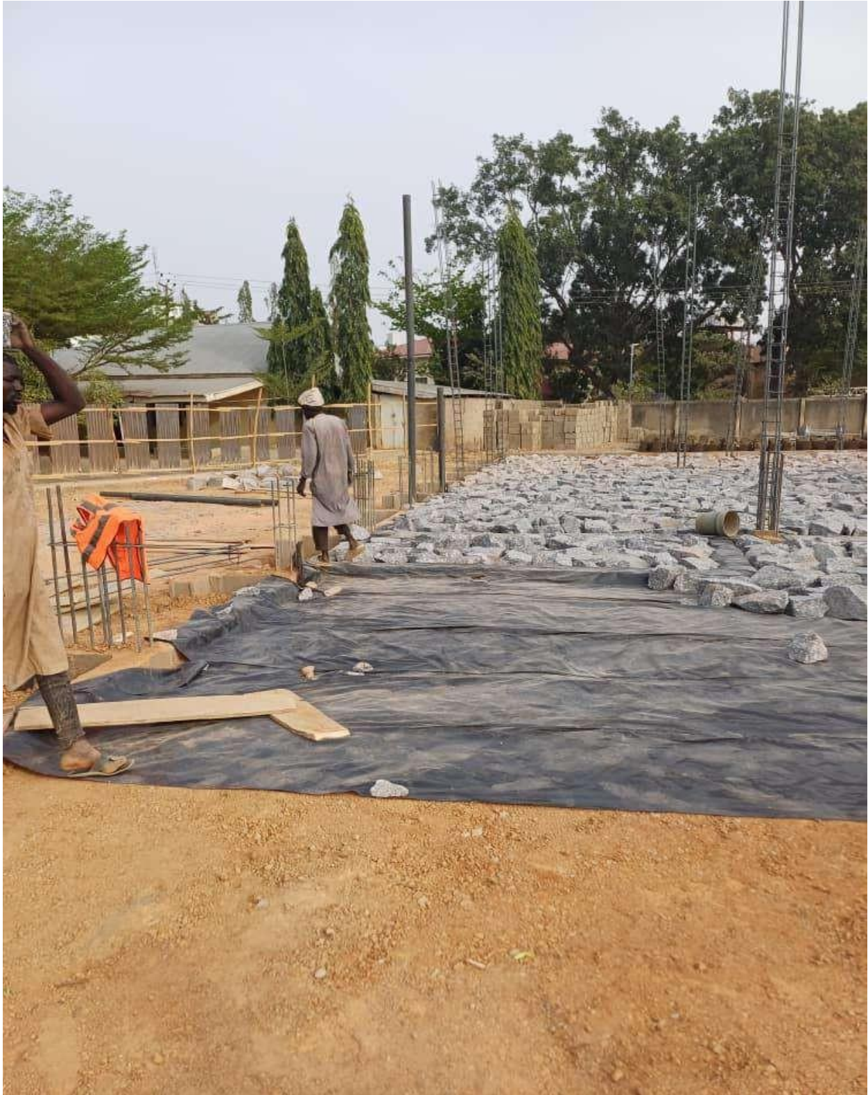
Laying of Damp Proof Membrane and Hardcore
