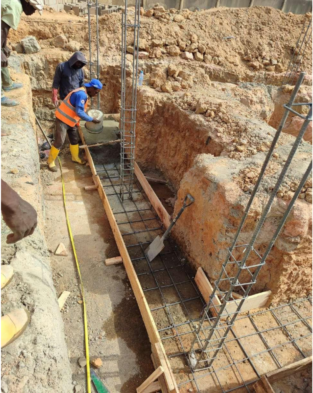
Formwork, reinforcement and concrete for reinforced Strip foundation
