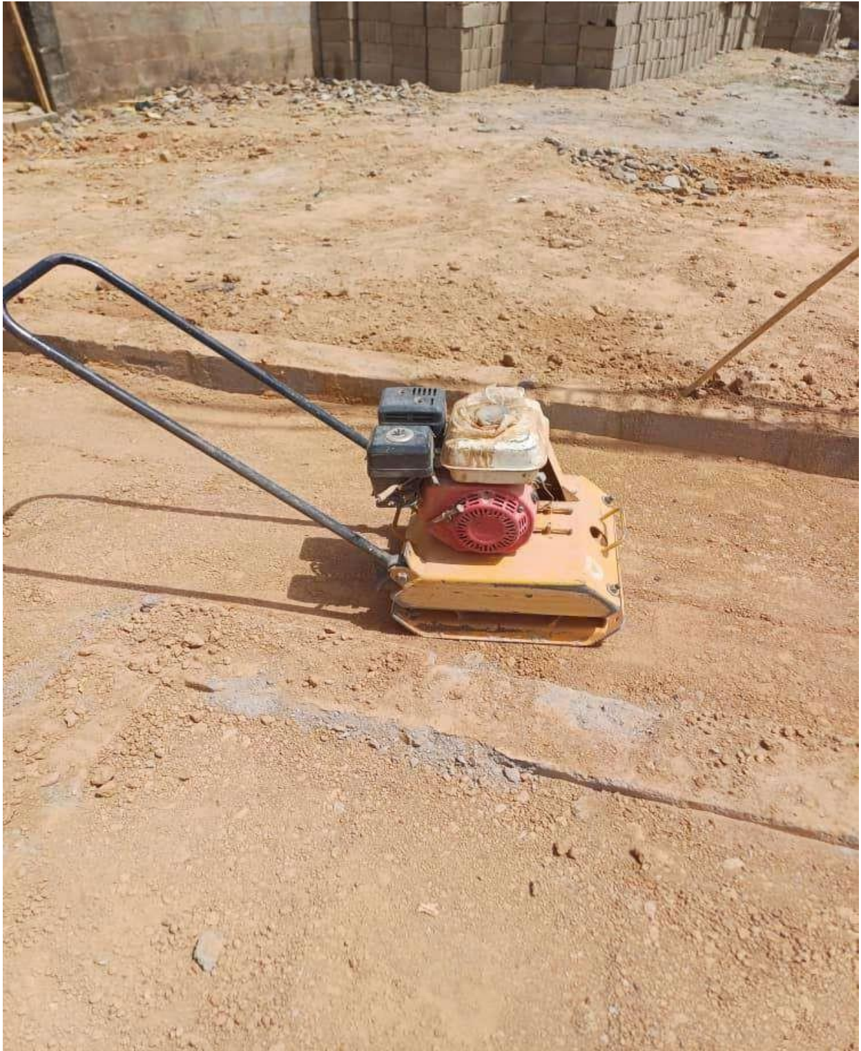
Compaction on going
