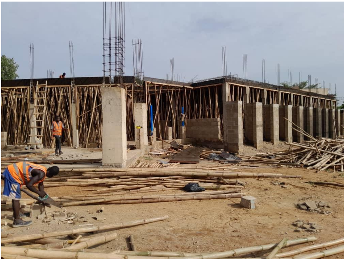
First floor slab formwork in progress 1
