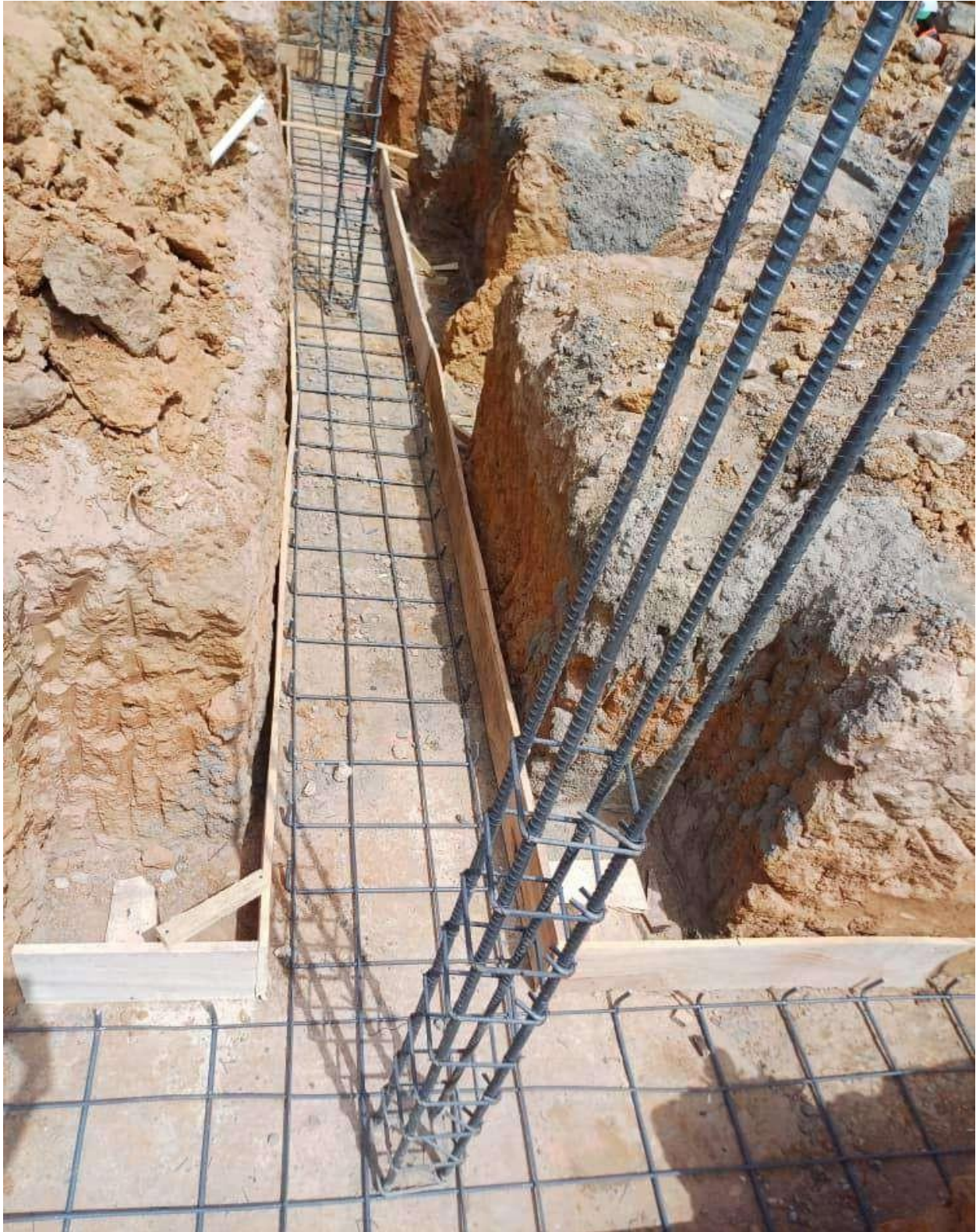
Formwork and reinforcement for reinforced strip foundation
