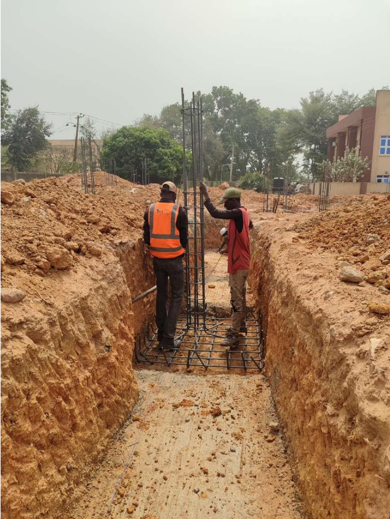
Reinforcement for bases and columns
