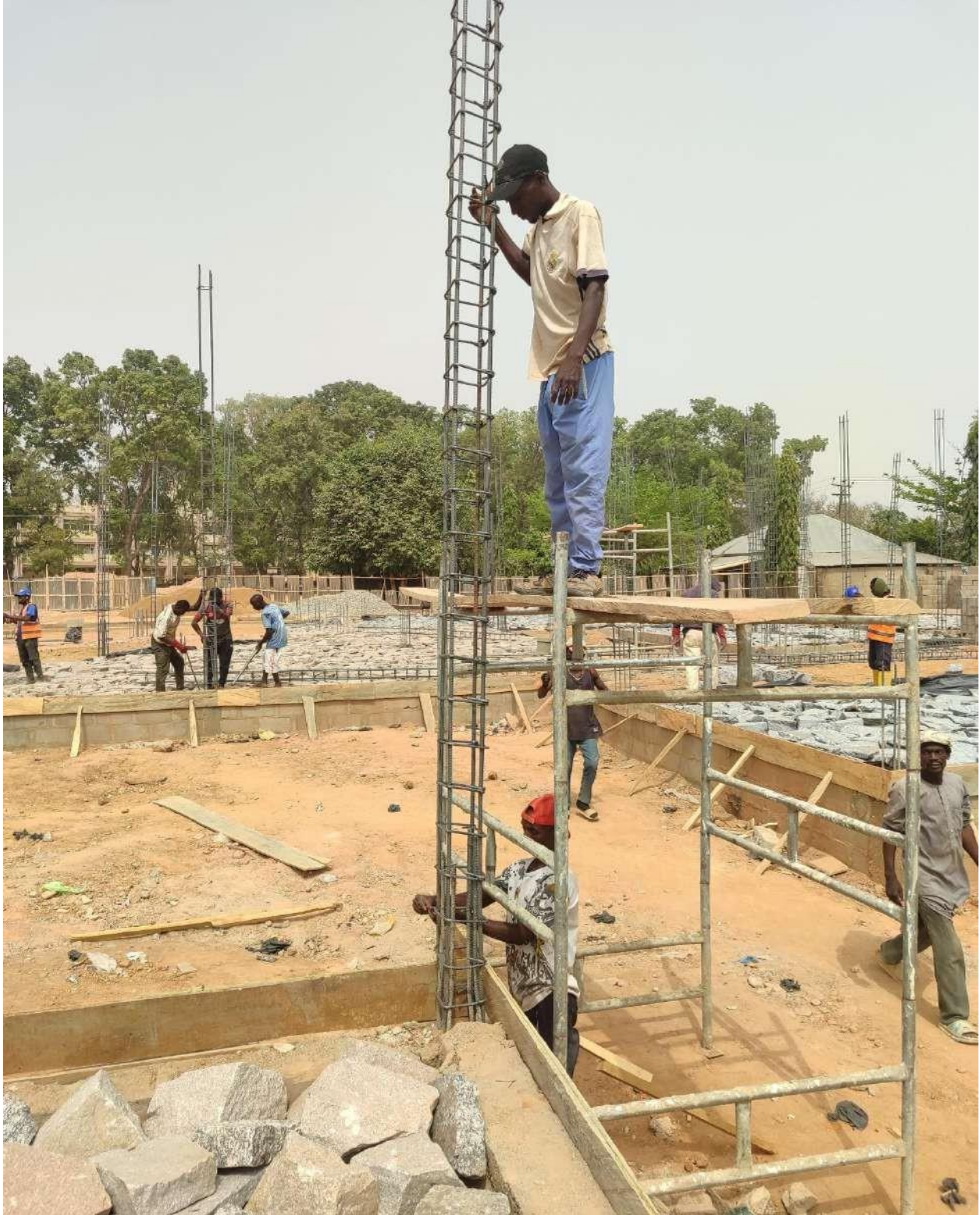
Erection of Column reinforcement
