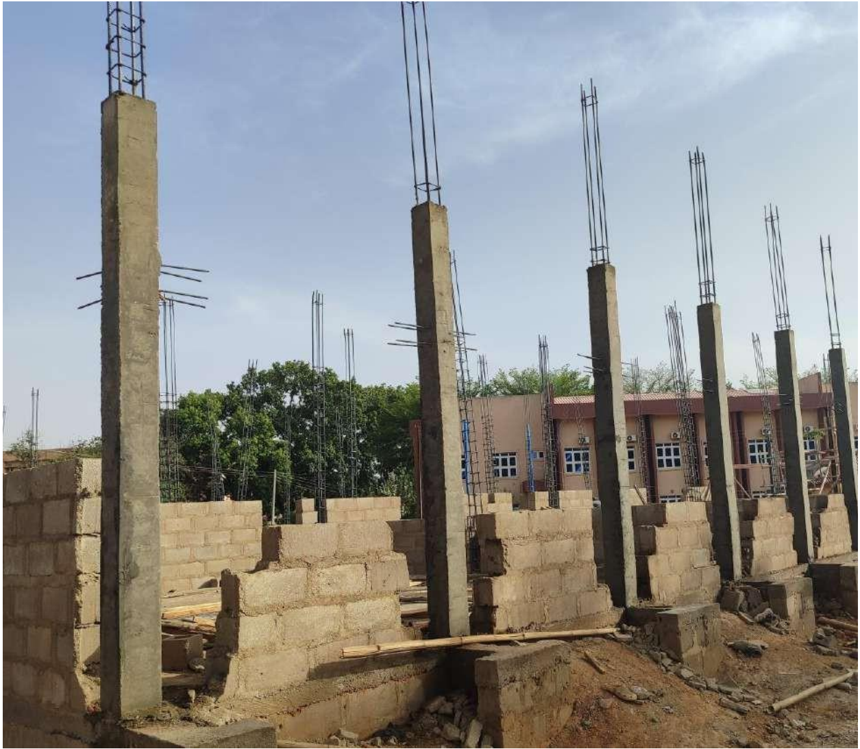
Columns after removal of formwork
