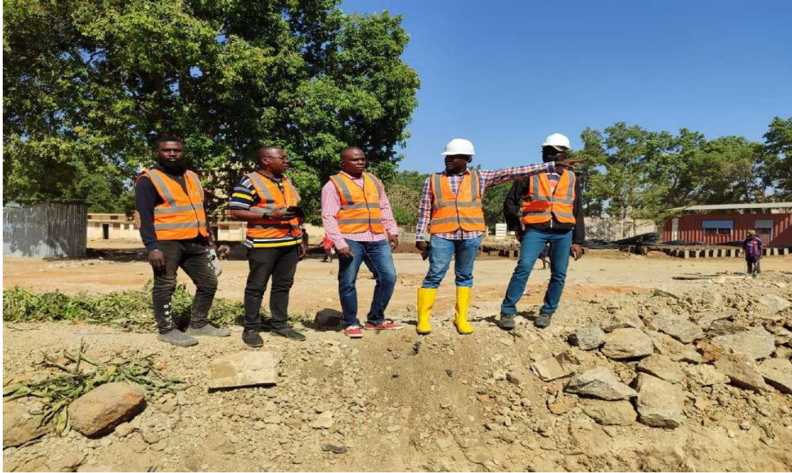
Consultants/contractors supervising excavation and earthworks
