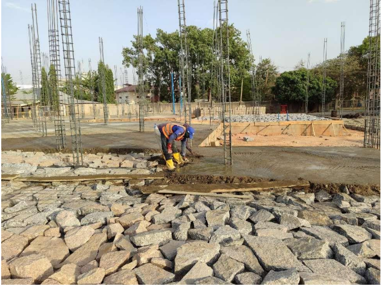
Casting of Concrete for DPC
