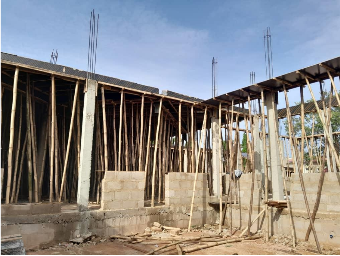
First floor slab formwork in progress 4
