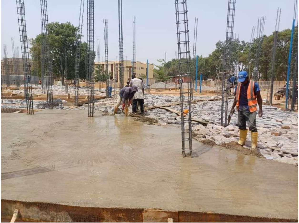
Casting of over site concrete in DPC
