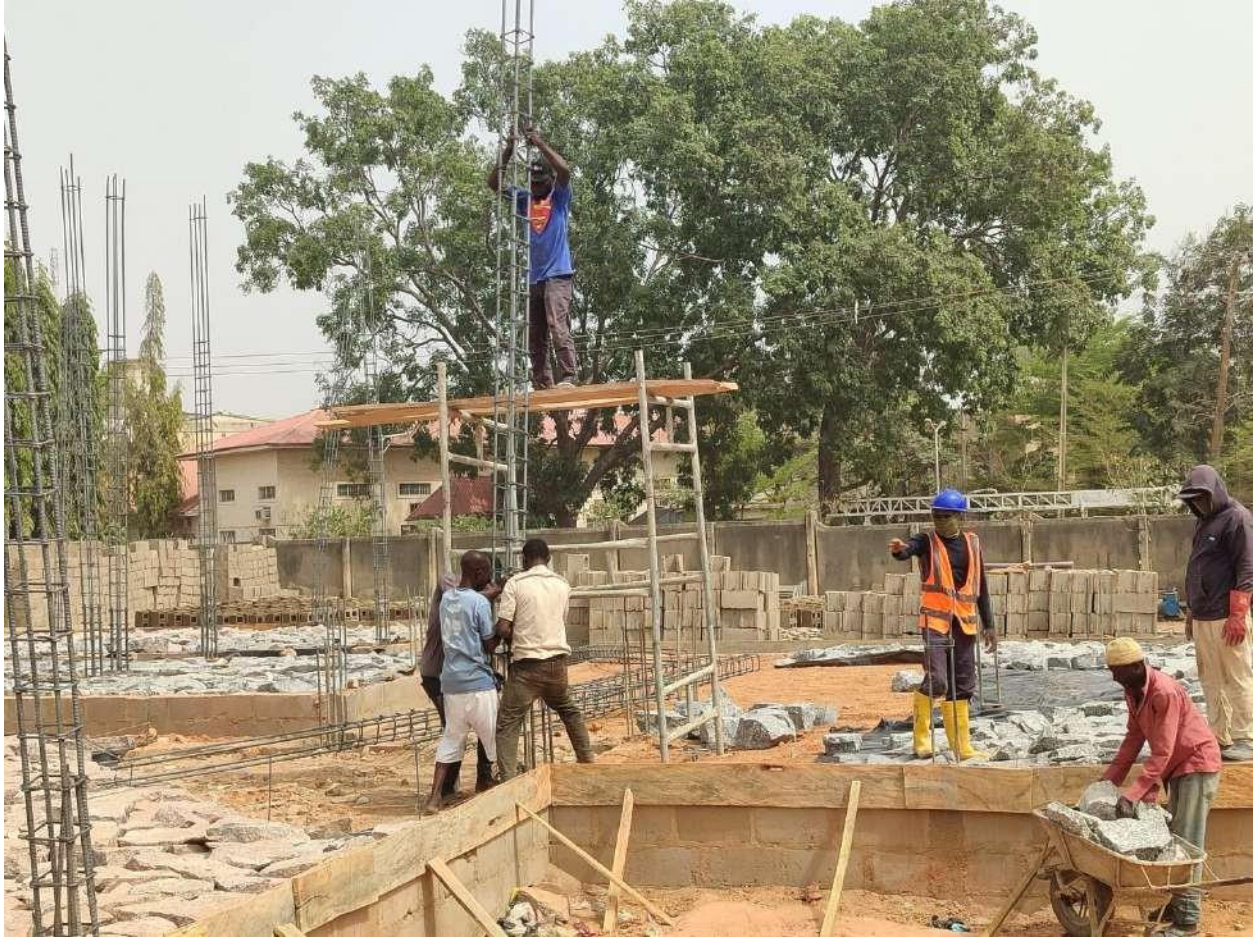
Erection of Column reinforcement
