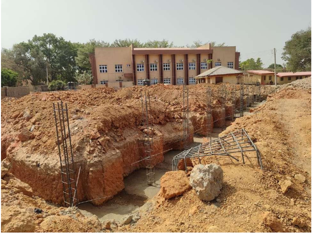
Concrete Base Casted and Short Column Standing
