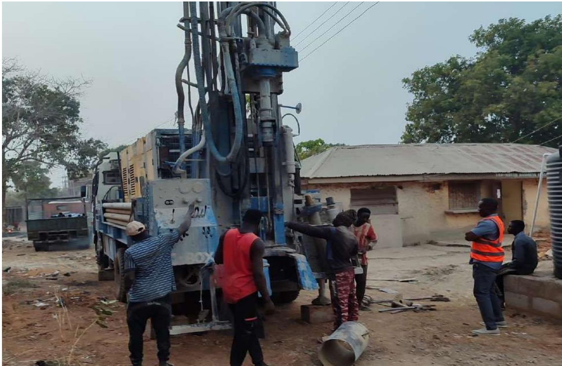
Geophysical survey and drilling of water borehole
