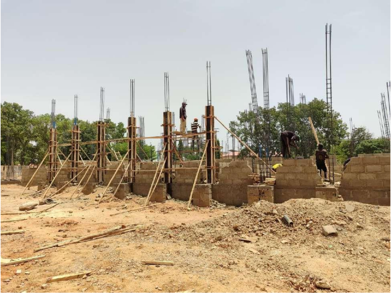
Form work for Column
