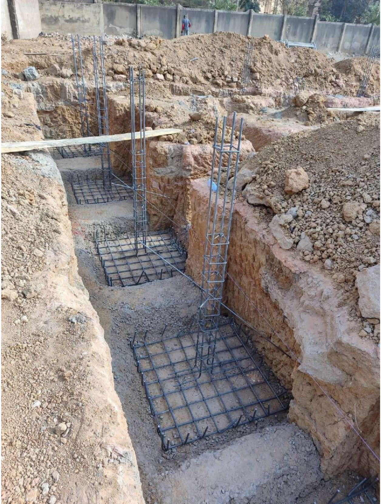
Reinforcement for bases and columns
