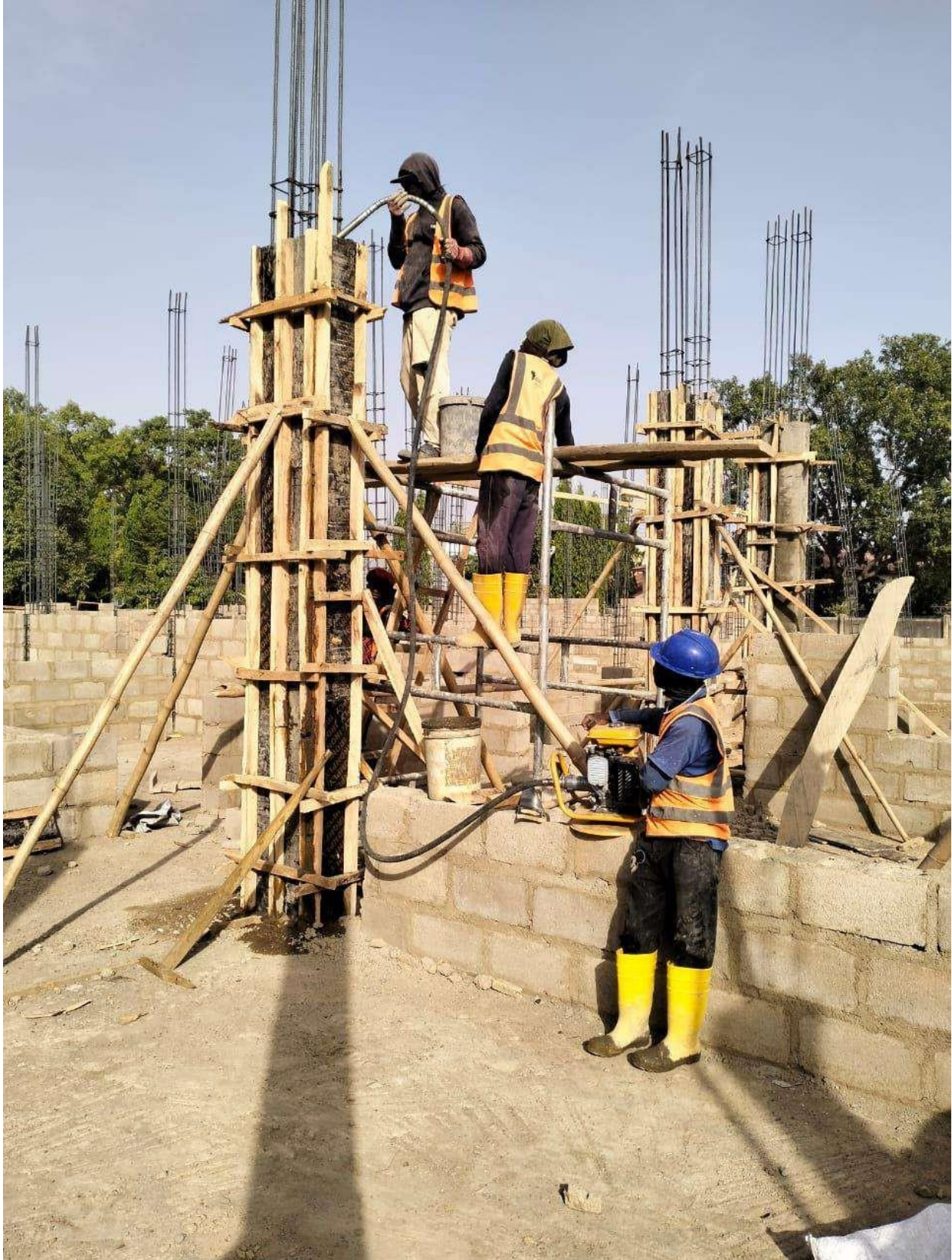
Pouring and compaction of concrete in Column
