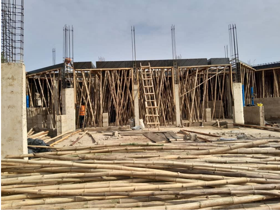
First floor slab formwork in progress 2
