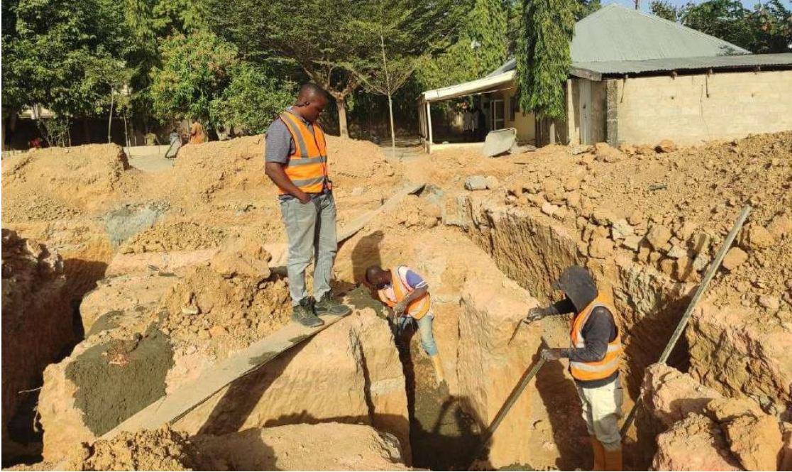
Blinding in progress 2
