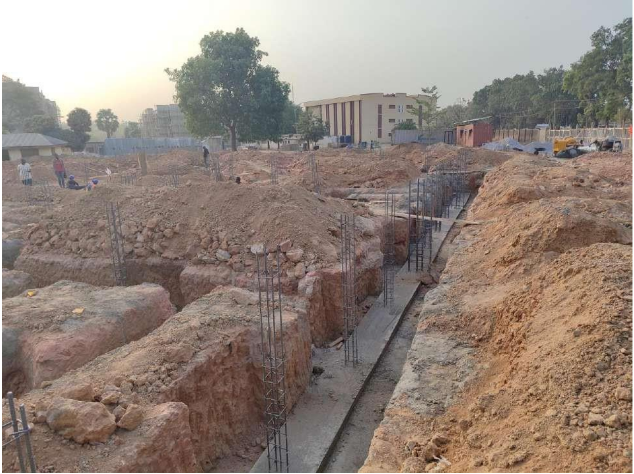
Reinforced Strip foundation completed
