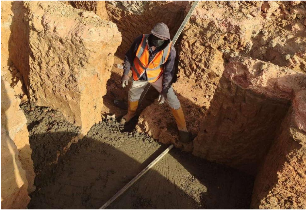
Blinding in progress 1
