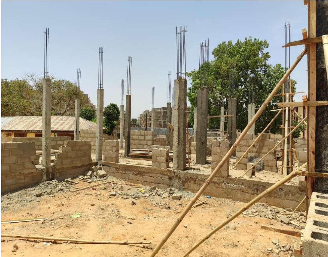
Columns after removal of formwork
