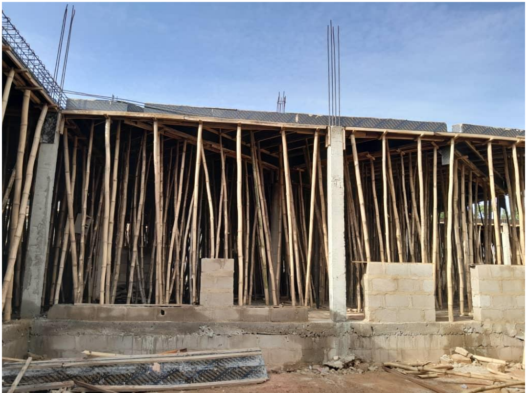
First floor slab formwork in progress 3
