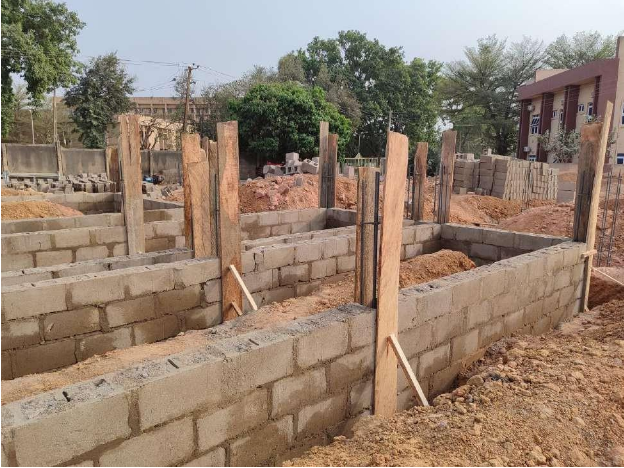
Formwork for columns
