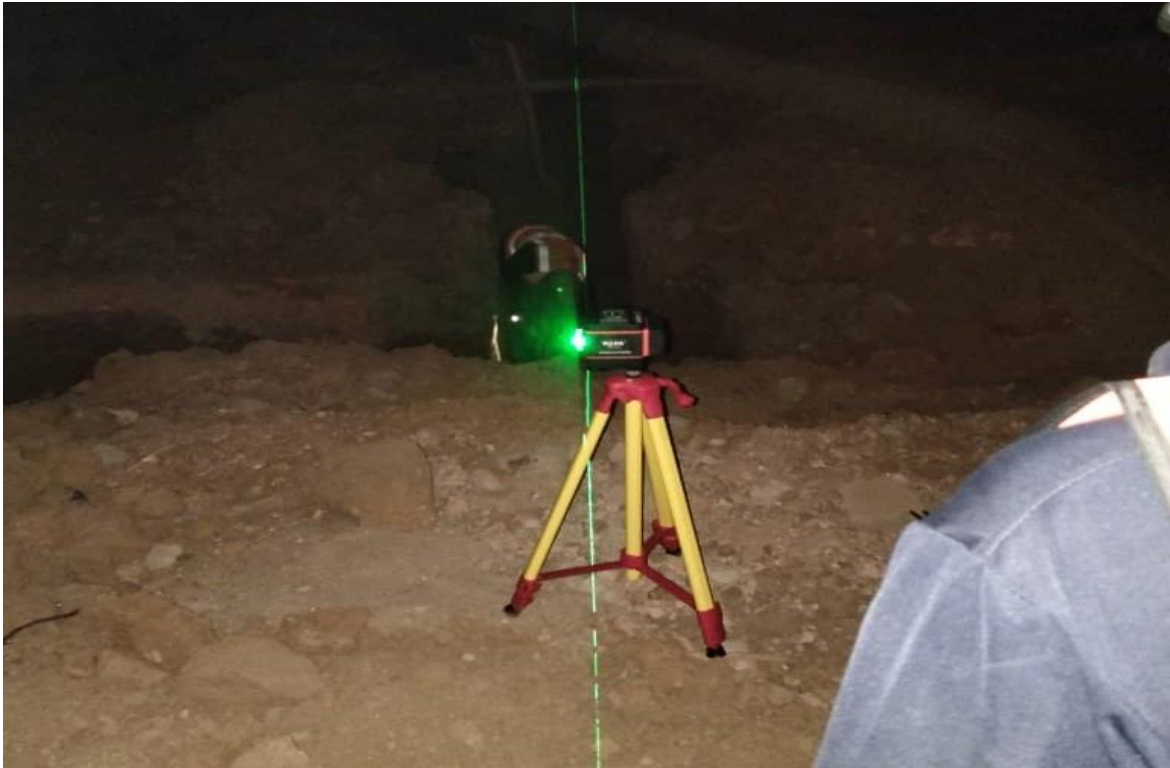
Levelling in progress
