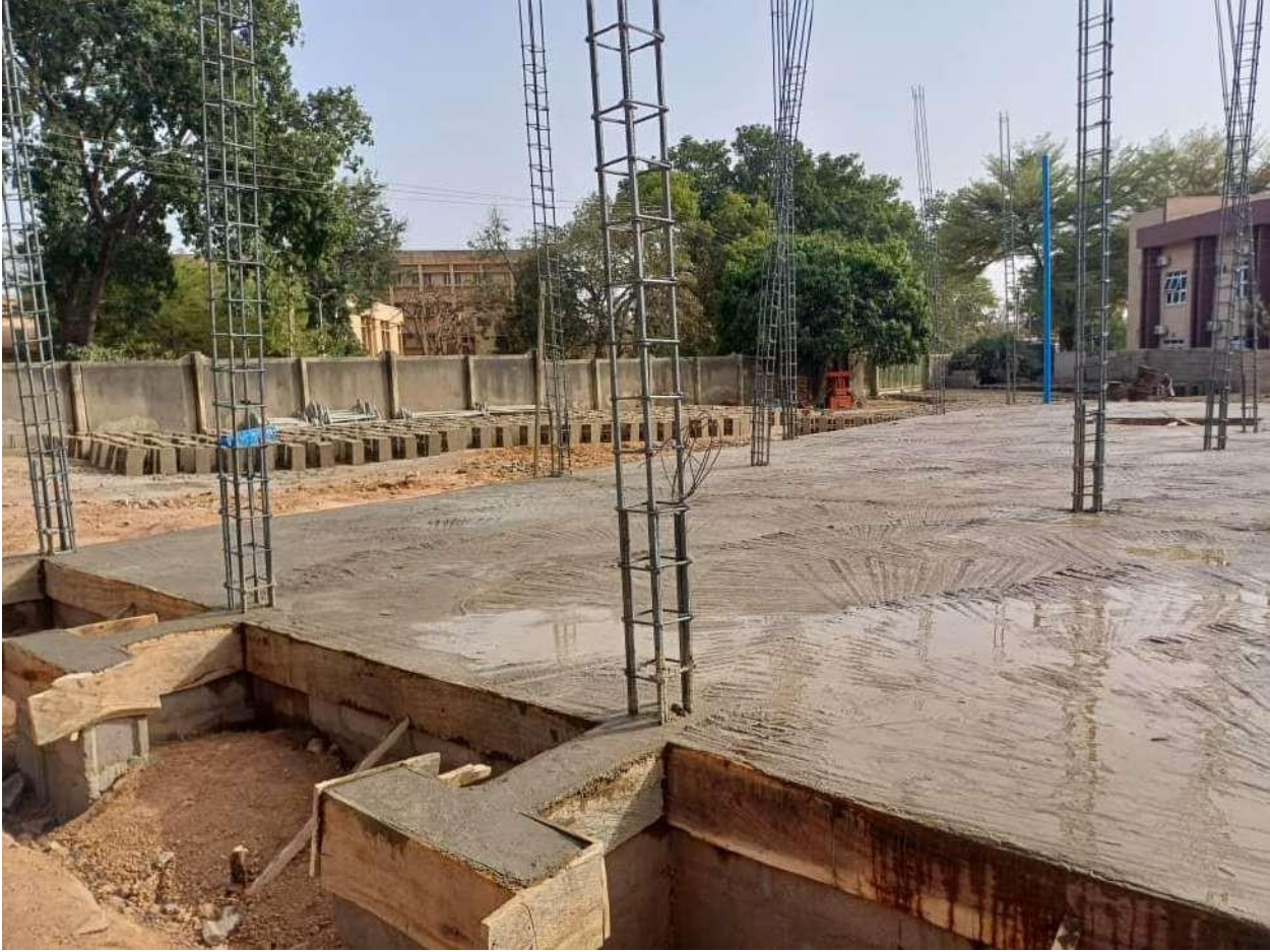
Curing of Completed section of Damp proof course
