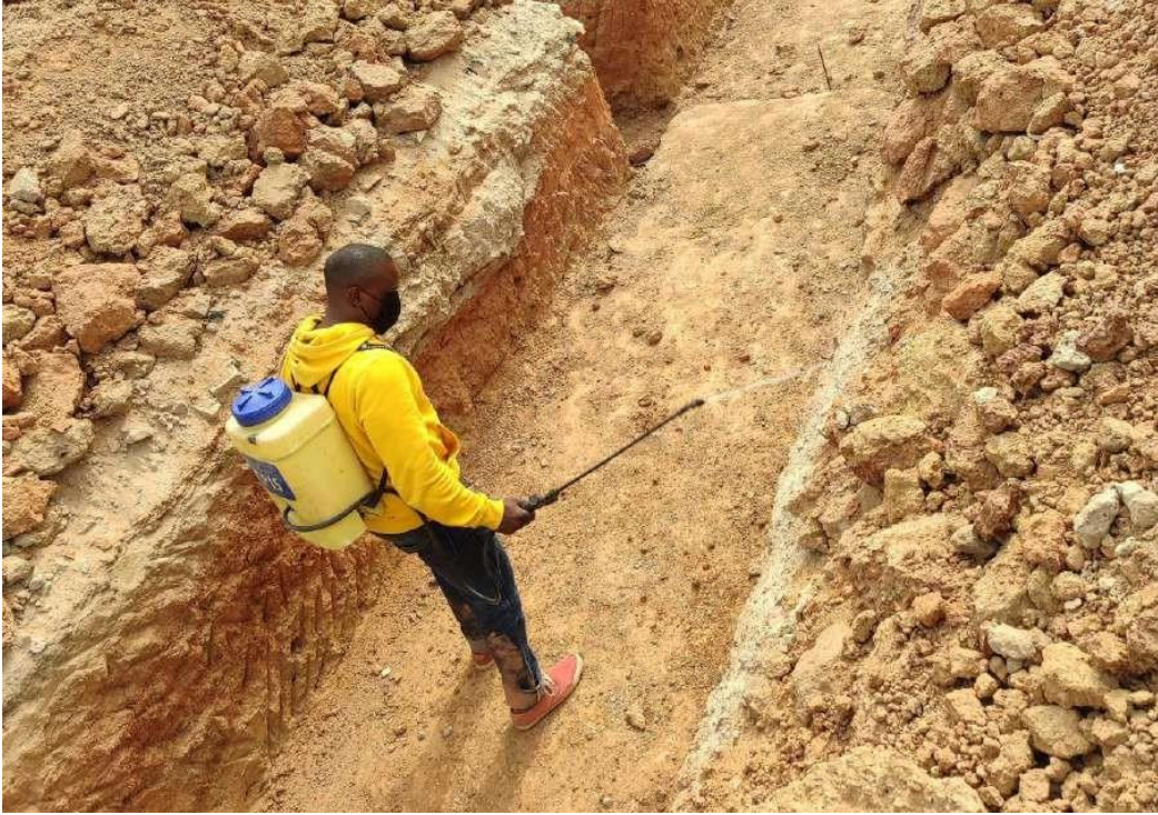
Anti-termite treatment to walls and bottom of excavation
