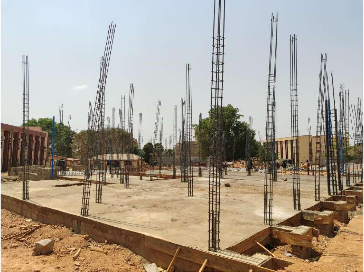
Completed Dam proof course
