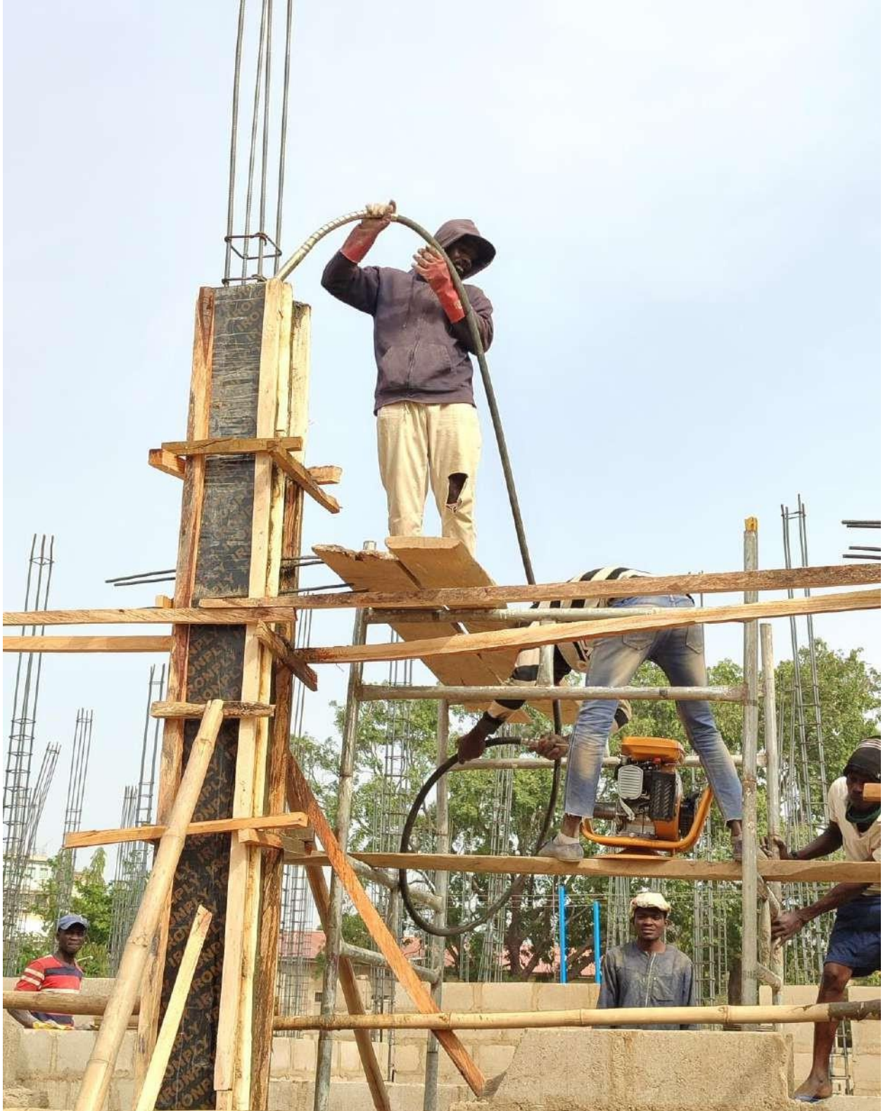
Pouring and compaction of concrete in Column
