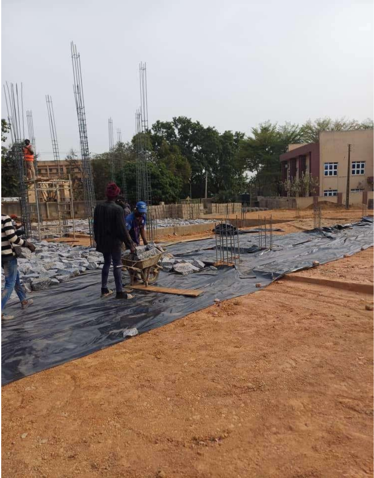
Laying of Damp Proof Membrane and Hardcore
