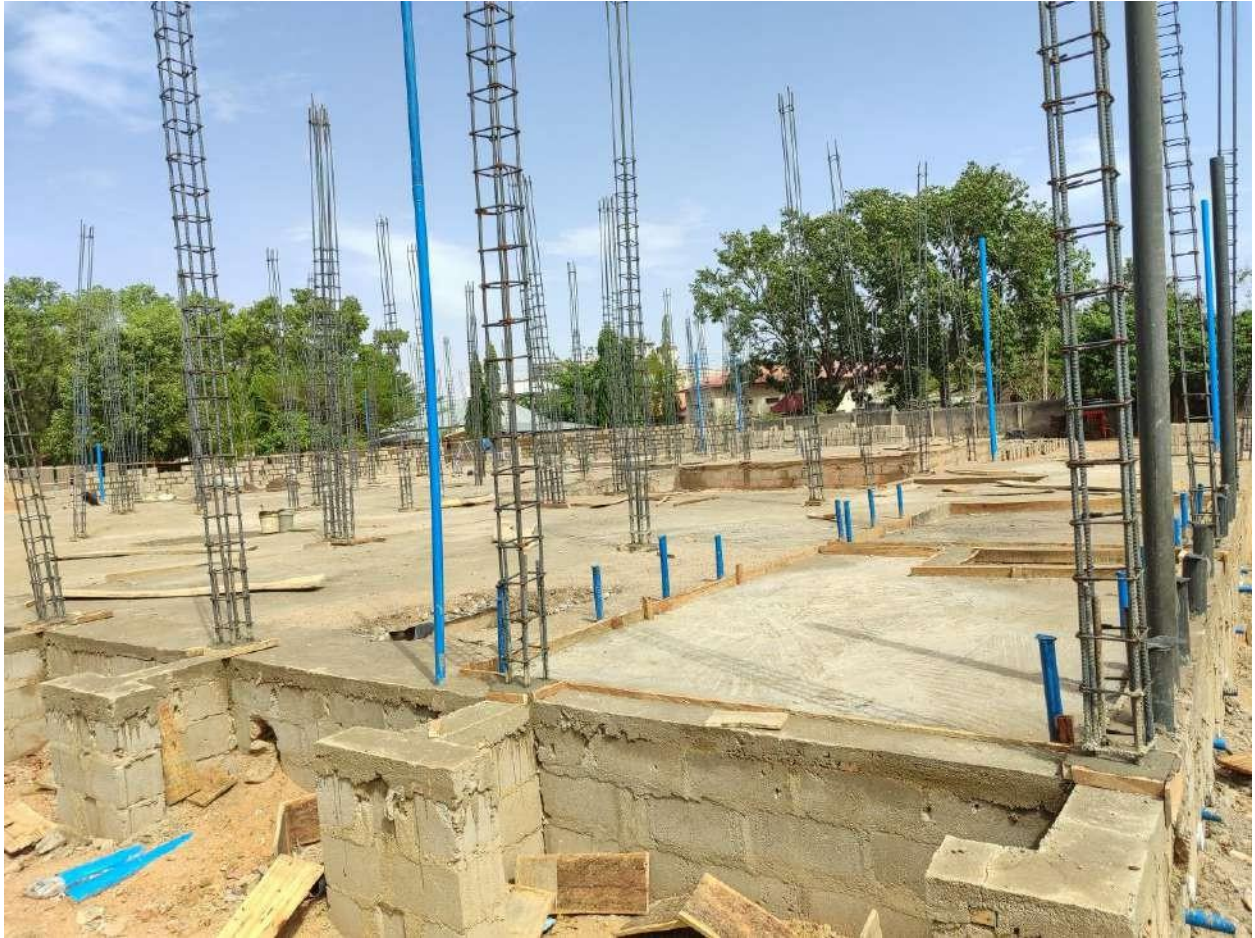
completed Damp Proof course
