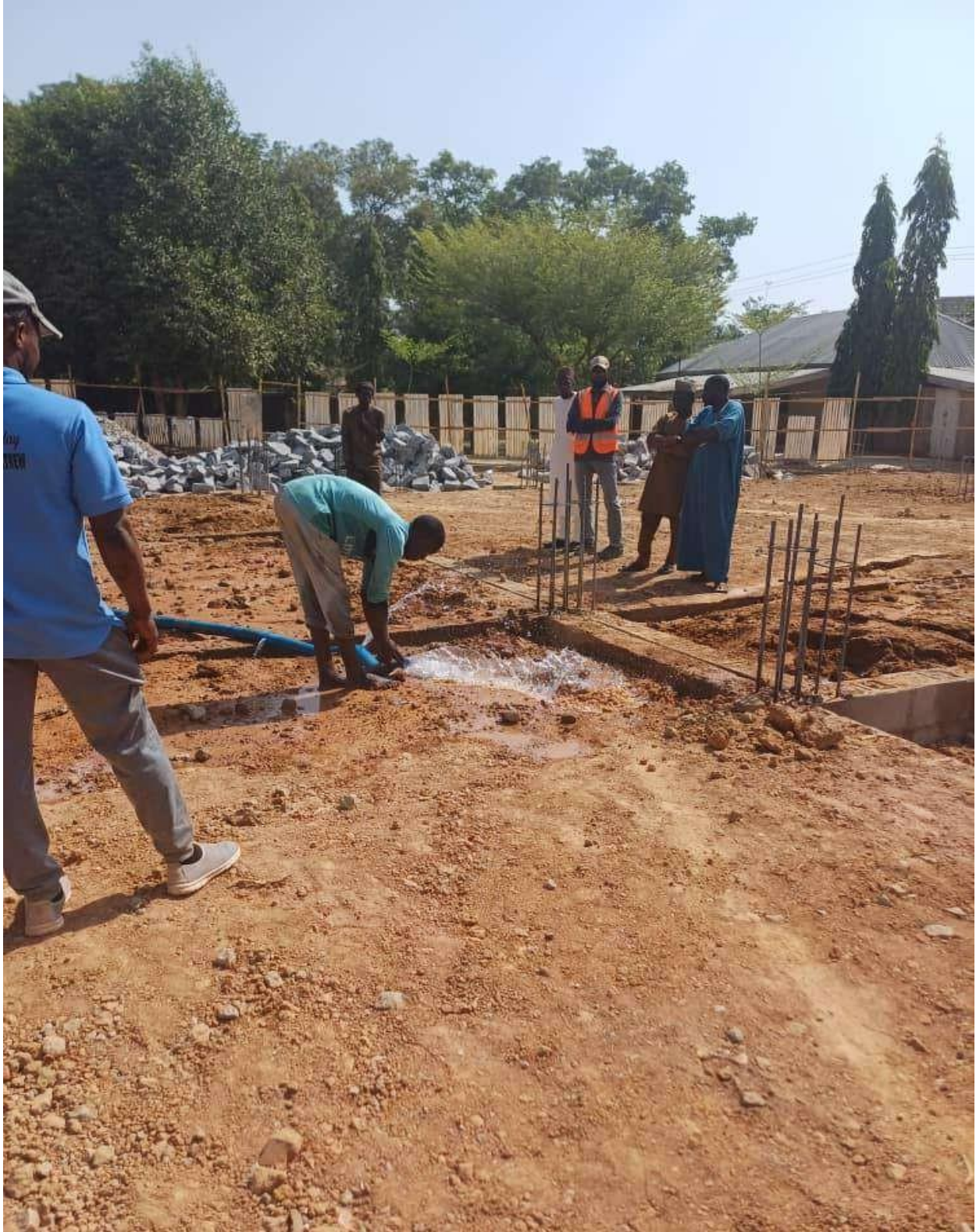
Watering after Backfilling for optimum soil compaction
