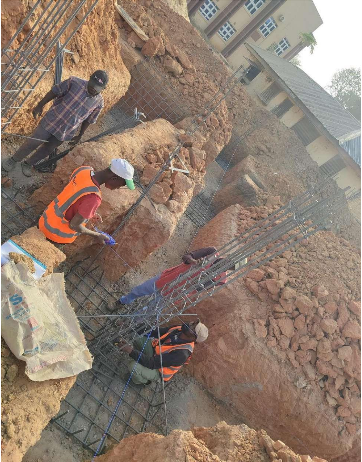
Setting of Column and Base Reinforcement
