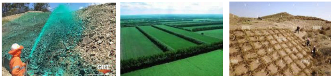
Plate III: (a) Chemical sand-fixing techniques (b) Agronomic techniques (c) Mechanical techniques (source: www.google.com)
